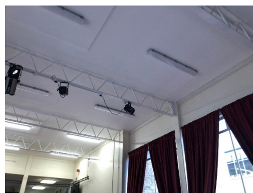
FIGURE 15 INTERNAL ROOF STRUCTURE HIGHFIELDS LOWER
