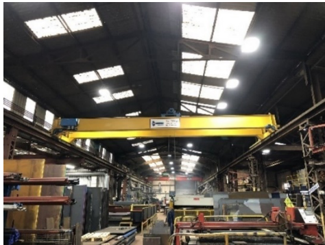
FIGURE 12 TWIGG STEELYARD INTERNAL ROOF STRUCTURE
