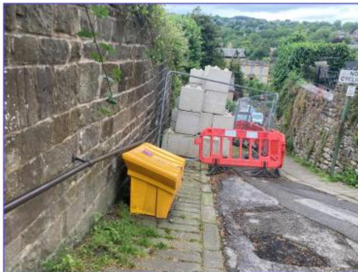
Figure 2 – Street view of the retaining wall, surrounded by temporary concrete barriers.
