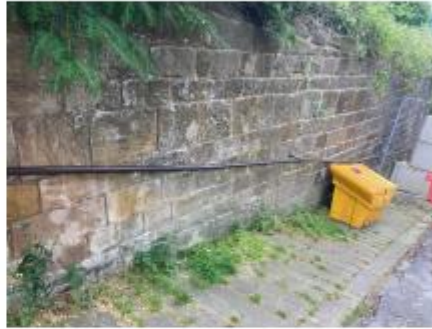
2.) Photograph showing retaining wall from the top of Stoney Way.
