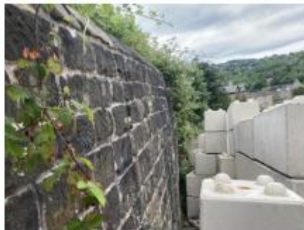
10.) Additional photograph showing retaining wall and the interlocking concrete blocks.
