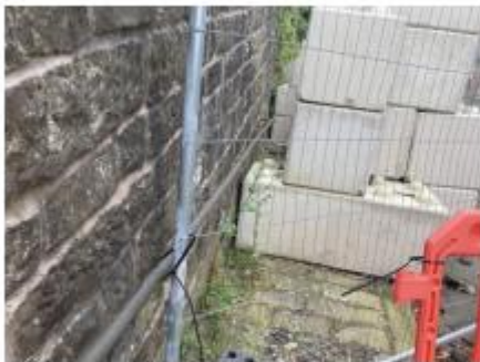
9.) Additional photograph showing retaining wall and the interlocking concrete blocks.
