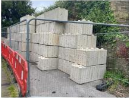
1.) Photograph showing interlocking concrete blocks providing protection in the event of wall failure.
